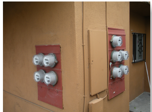
Electric Service Panel
