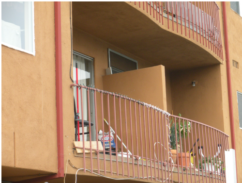
View of Balcony
