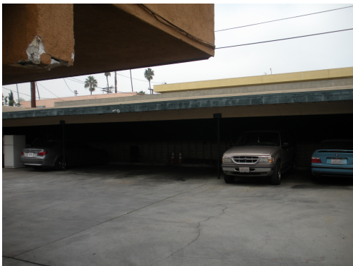
Carport in rear
