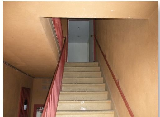
Stairwell to Upper units
